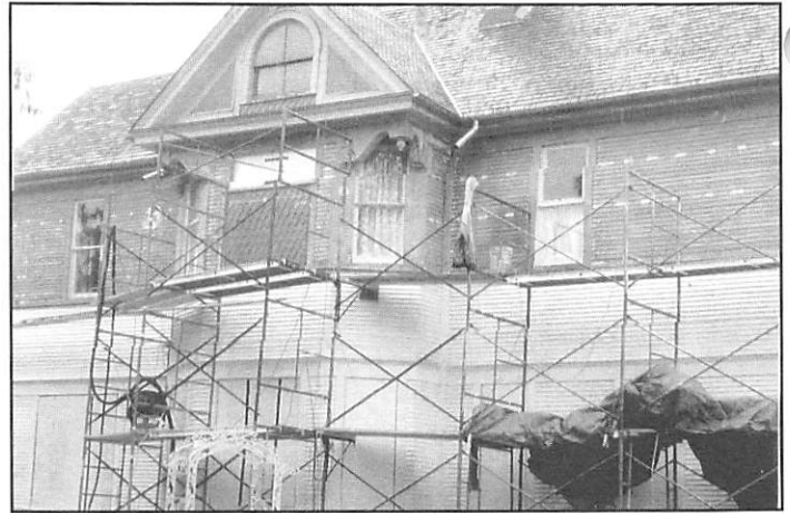
Exterior restoration on the east side of Elmwood.
