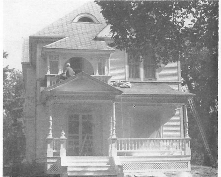
Historic Elmwood with new porch.
