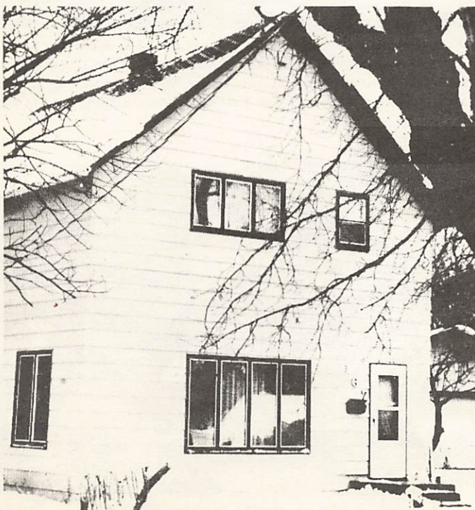
The Cooper house as it looks at the present time, with the extensive remodeling done by the current owners, Bill and Rosemary Rodgers.
