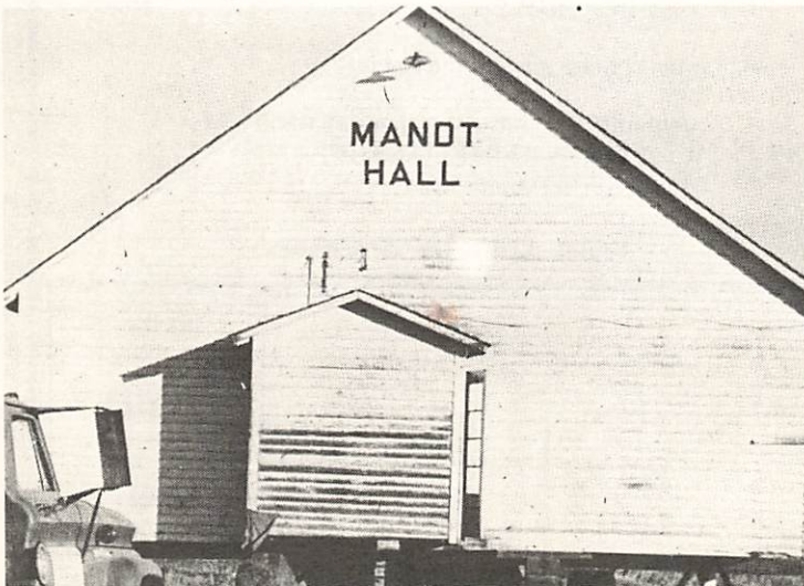
The old Mandt Hall from west of Grafton was moved to the Village grounds on November 12. The building was owned by Harvey Tallackson, who donated it to the Village. A group of Mandt area people are paying the moving expenses and The Grafton Record will provide a cement slab for the hall and will refurbish the building. The Record plans to use part of the building for an old time print shop display and remainder of the building will be available for other displays.
